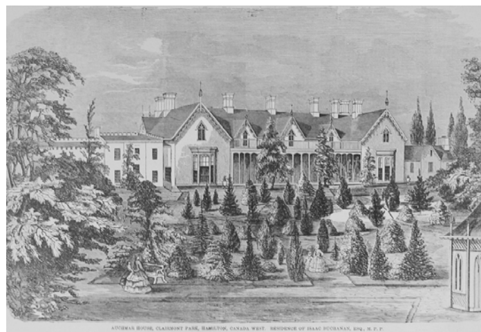
Etching of the North Elevation. This image includes the kitchen wing along with a west wing (to the right of the image) and octagonal garden pavilion that no longer exist.
